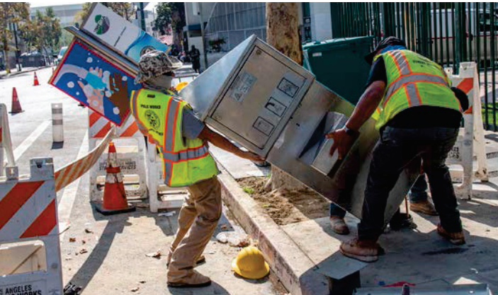
Washing/Hydration Station Installation in Skid Row
